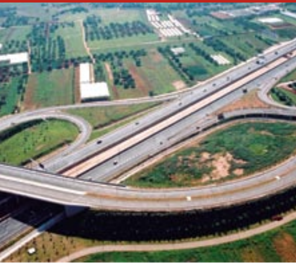
Aerial view of the Attiki Odos Motorway heading away from the airport.
