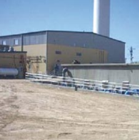
Webb County Water Treatment Plant in Rio Bravo, Texas
