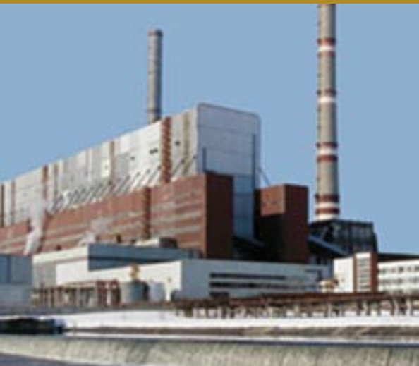
Permskaya Gres power plant in Dobryanka, Russia
