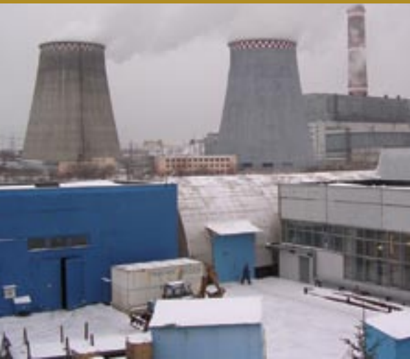
Main Plant at Mosenergo Heating and Pipeline in Moscow, Russia
