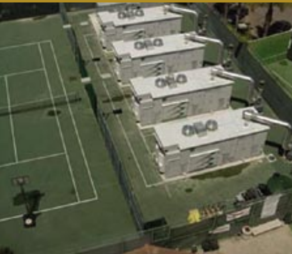
Fuel Cell Energy DFC 300s on a San Diego, CA tennis court
