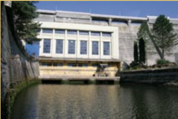
An E.ON Hydroelectric Power Plant
