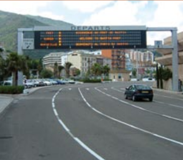
A Signature S.A.-created road sign in France
