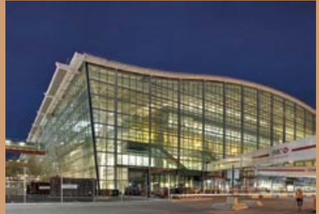
Heathrow Airport's T5 Terminal
