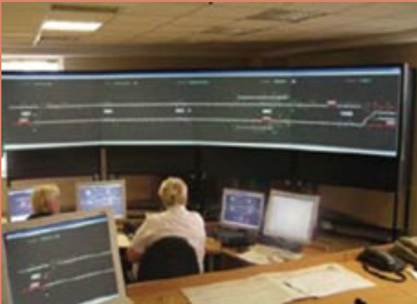
Dispatching Desk at Kazan Metro Operations
