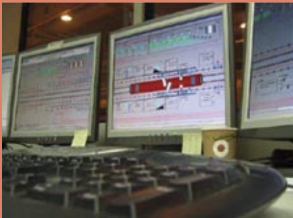
Train Wash Operator Control Area
